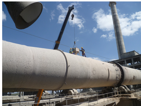
FIGURE 2. Direct feeding of the clay to the rotary kiln.
