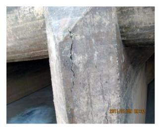
FIGURE 1. An example of freeze-thaw damage of a dam sluice.
