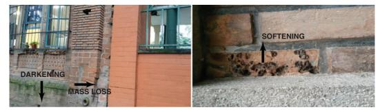
FIGURE 3. Stone structure degradation caused by external agents. The structures displayed mass loss and darkening. Universidad Nacional de Colombia at Medellin. Left: sample 3 and 4; Right: sample 5. (see table 2) (Photos: E. Mejia).
