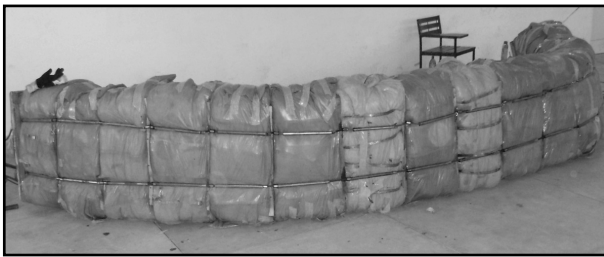
Figure 11. Pre-stressing for fabrication of Arch.
