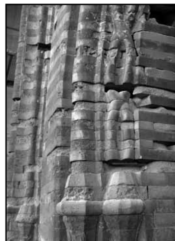
Figura 2. Detalle de la portada. Figure 2. Portal detail.
