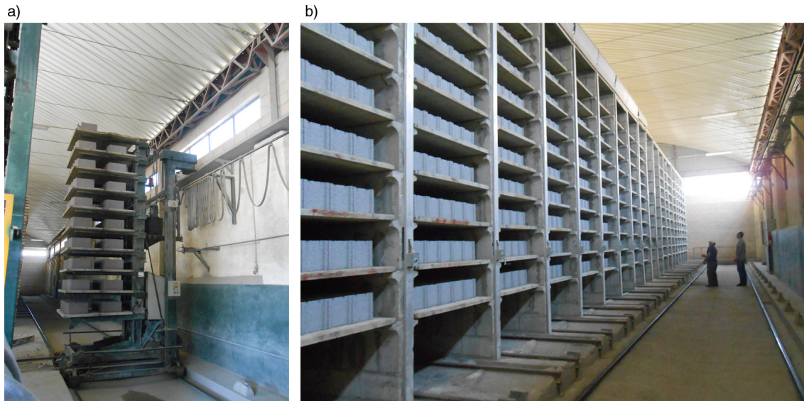
FIGURE 3. Manufacturing of CMU-PCC – Curing/drying: a) automatic transportation and b) curing chamber.
