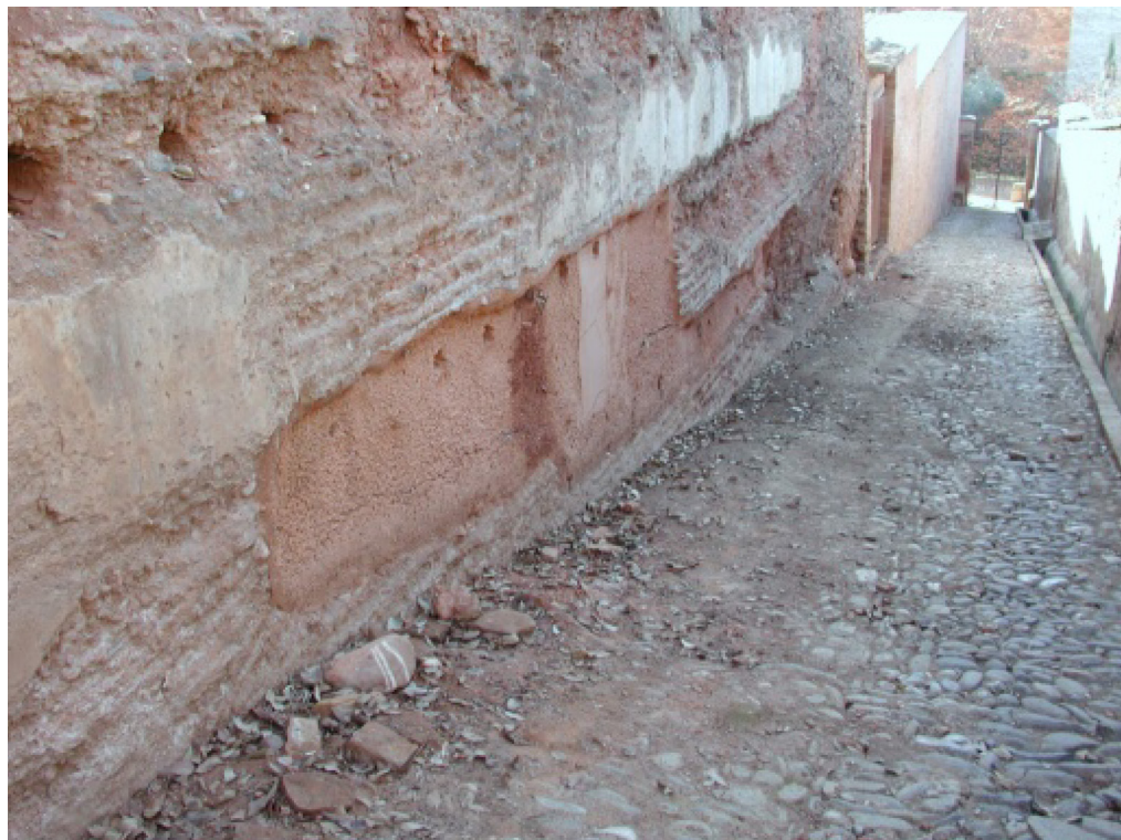
FIGURE 6. Restoration of a rammed earth wall with significant loss of mass at the base.
