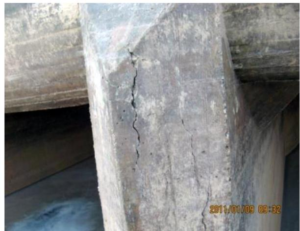
FIGURE 1. An example of freeze-thaw damage of a dam sluice.
