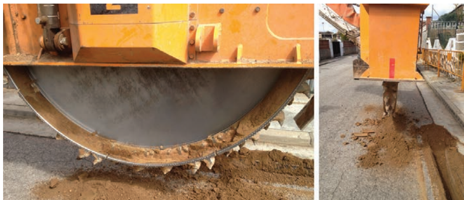
FIGURE 2. Excavation of a narrow trench and trench arisings.
