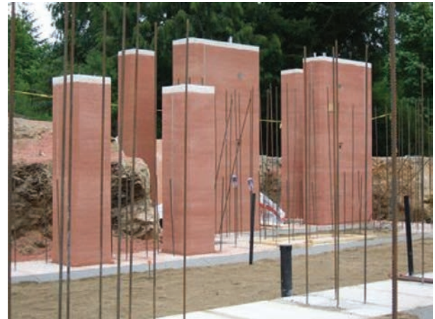
FIGURE 1. Steel reinforced rammed earth columns (Source: Clifton, 2015).
