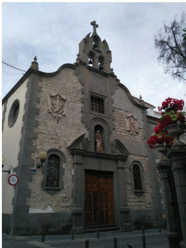
FIGURE 2. Historic building with unprotected wall surface of tuff stone.
