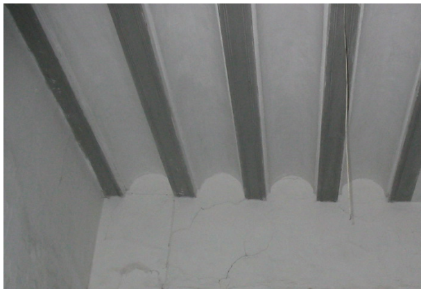
FIGURE 15. Section and picture of jack arch slab.
