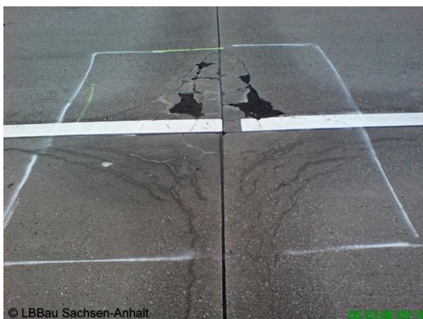
FIGURE 1. Example of an ASR-damaged highway pavement section with typical crack pattern and discolorations around the joints, especially at the cross points.
