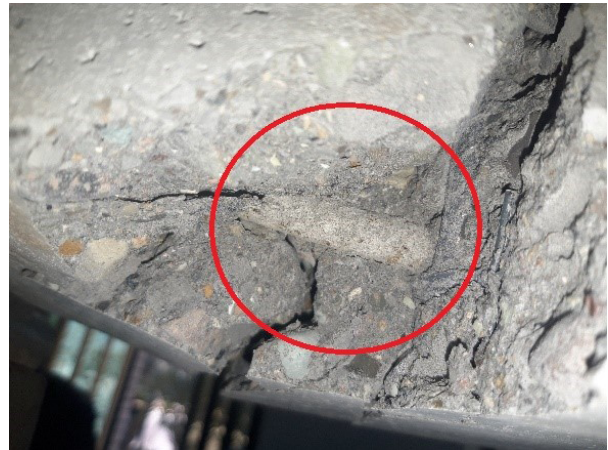
FIGURE 19. SGFRP rebar in concrete beam after loading.
