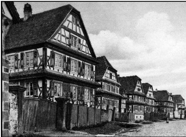
Figure 13. The colombage building type made of timber framed masonry or plaster (24).
